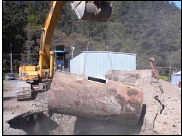
Excavating a leaking UST (LUST) and preparing the cavity for soil sampling.
