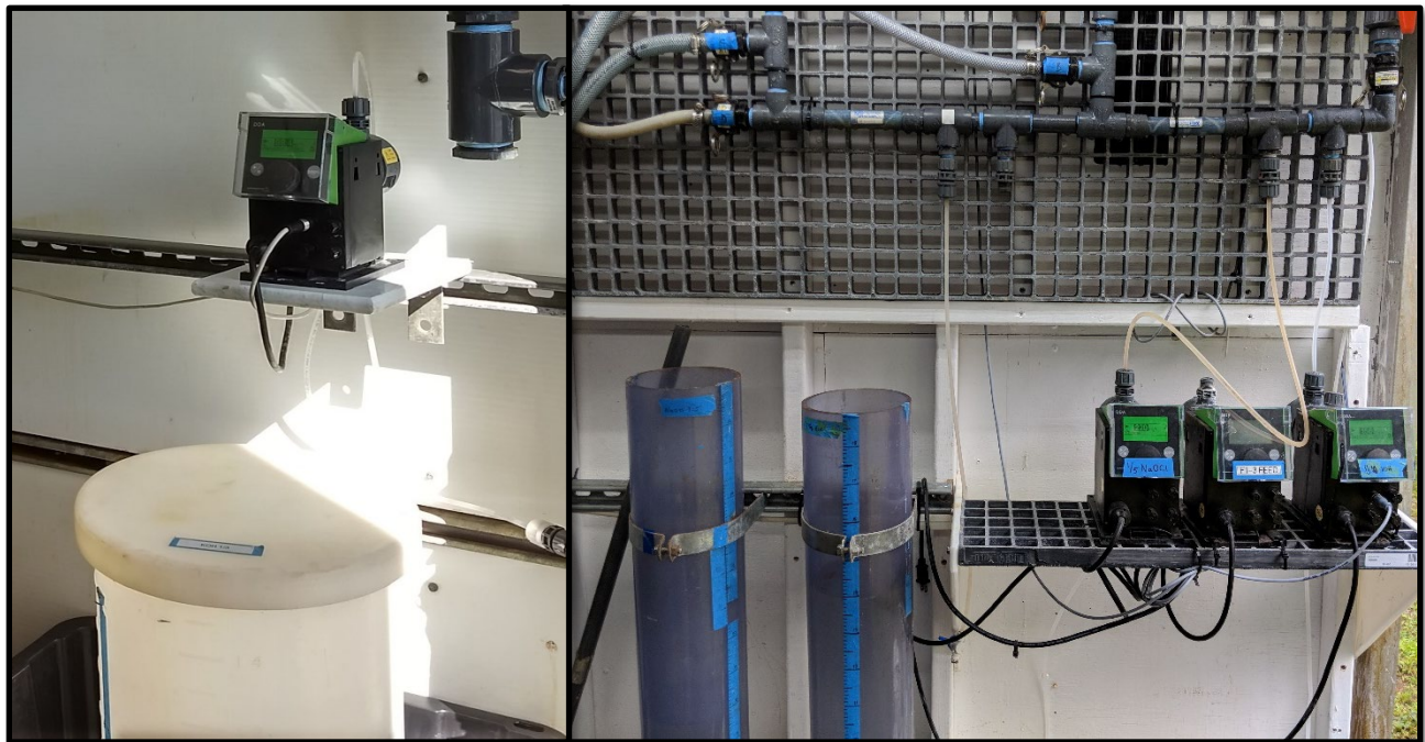
Figure 2.21: Pretreatment Chemicals in the Biological Pilot (Left) and the Greensand Pilot (Right)
