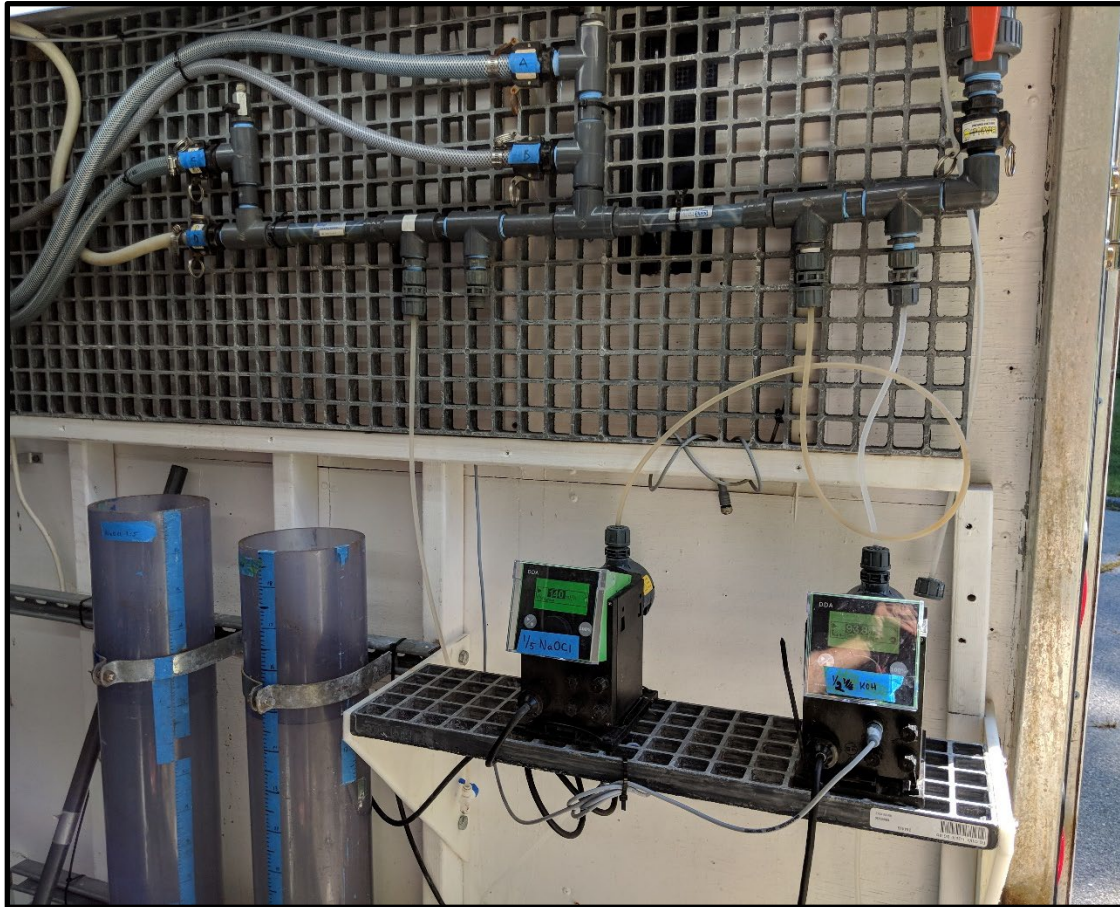
Figure 2.06: Pilot Trailer Chemical Feed Area
