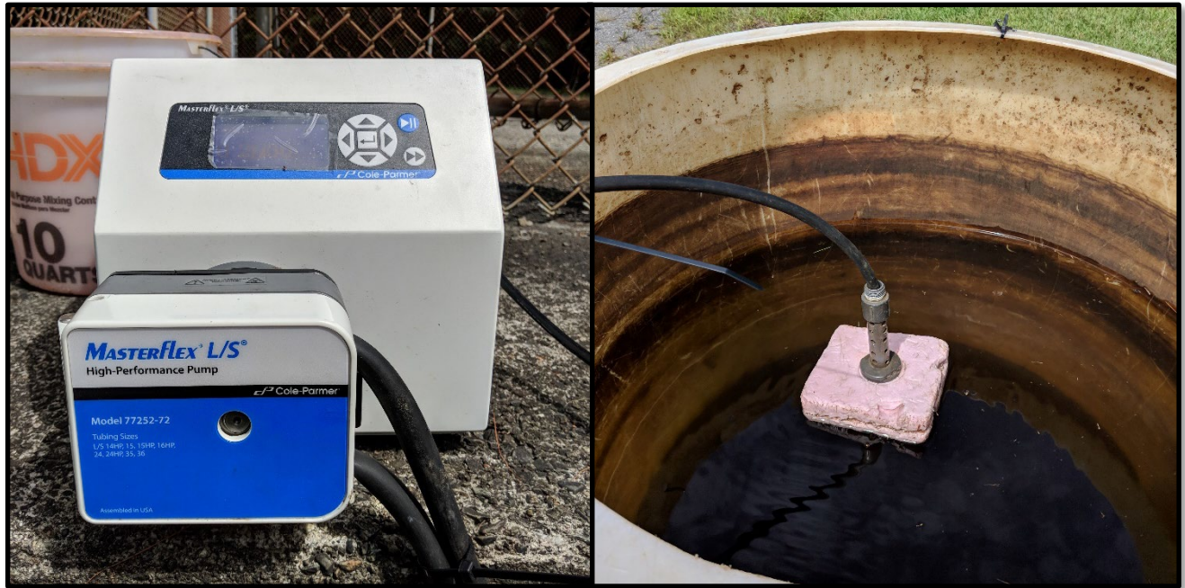
Figure 2.10: Supernatant Recycle Pump and Intake
