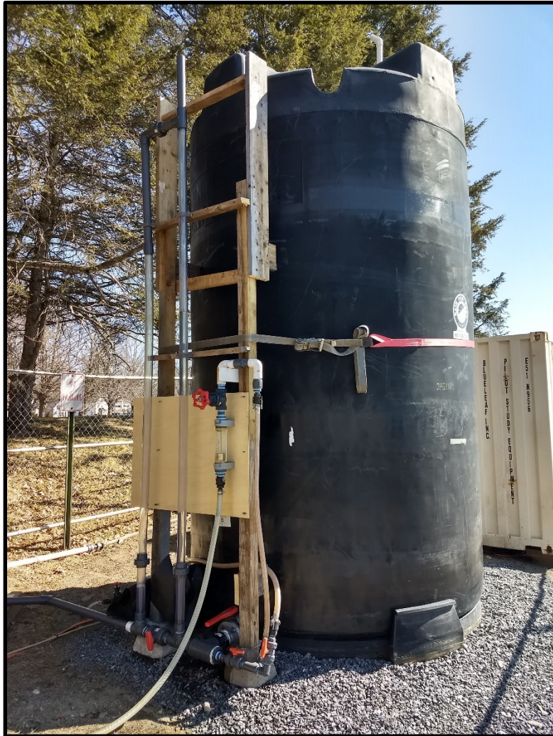
Figure 2.02: Raw Water Storage Tank
