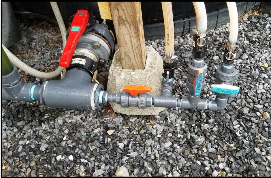
Figure 2.03: Raw Water Feed to Pilot Systems
