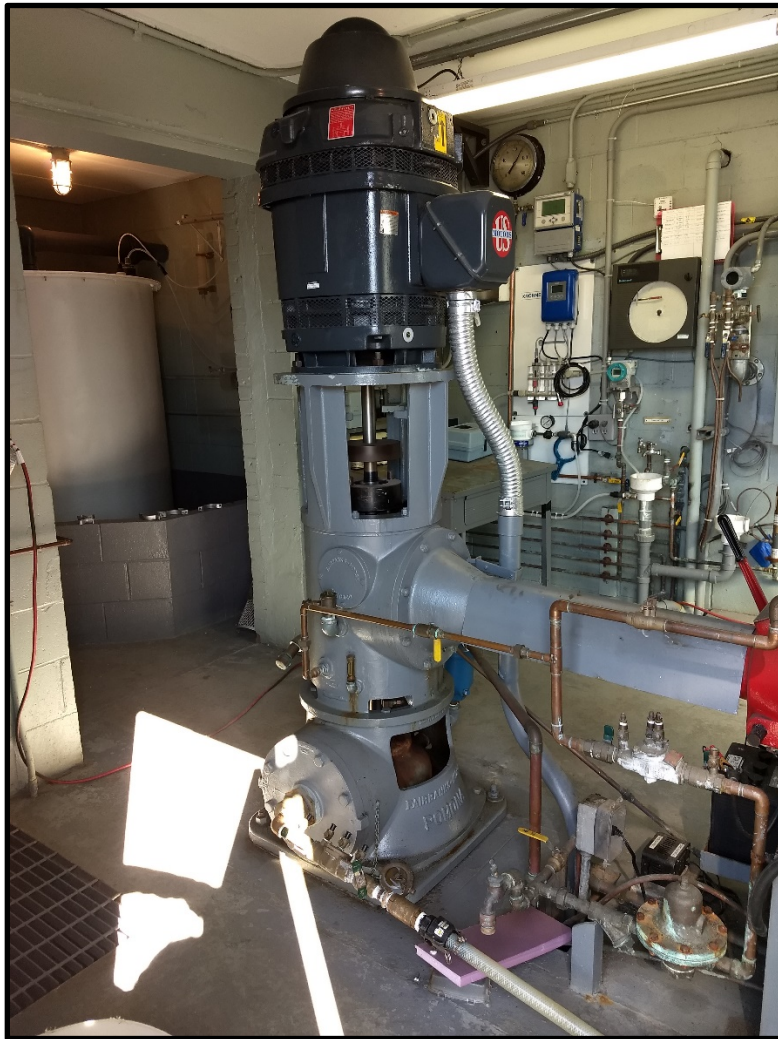
Figure 2.01: Oakdale Well Pilot Connection
