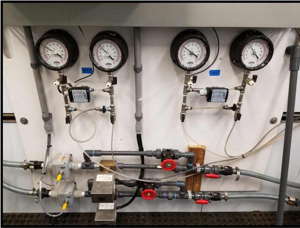
Figure 2.17: Flow Controls for Filters
