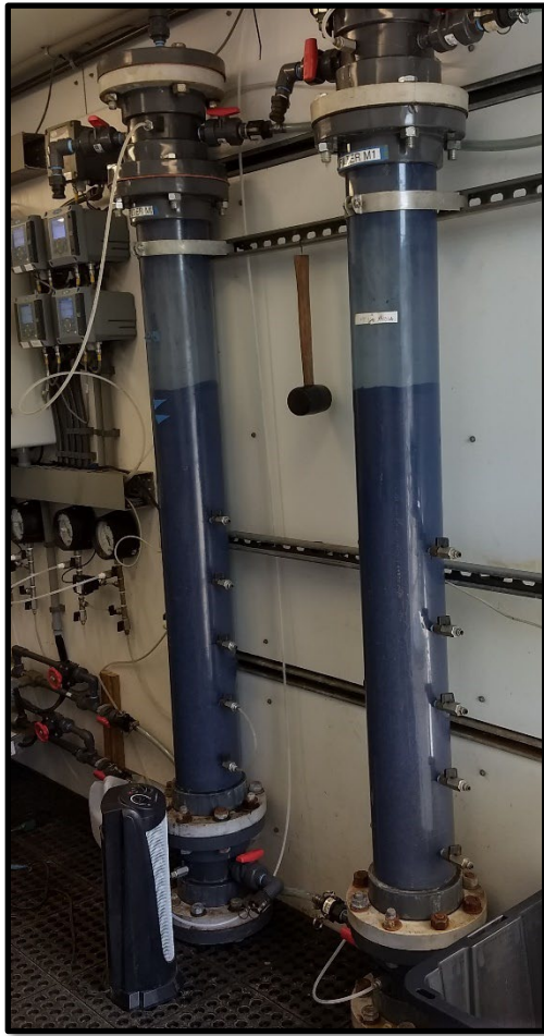
Figure 2.15: Filter Vessel M1 and M2
